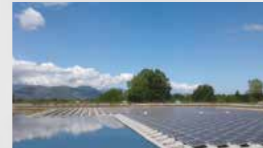
PONTECORVO, ITALY - 343 kWp
