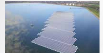
QE2, UK - 6,338 kWp
