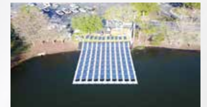
ORLANDO UTILITIES, USA - 32 kWp
