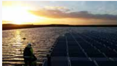
POLYBELL, UK - 471 kWp
