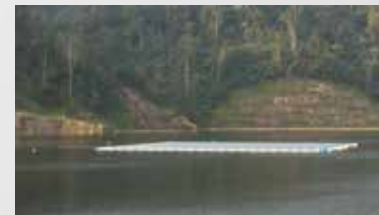
ULU SEPRI, MALAYSIA - 270 kWp
