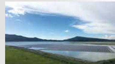
AGONGDIAN, TAIWAN - 2,320 kWp
