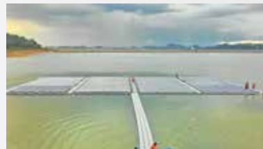
SUNGAI LABU, MALAYSIA - 108 kWp
