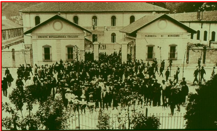
The plant in 1915 ...
